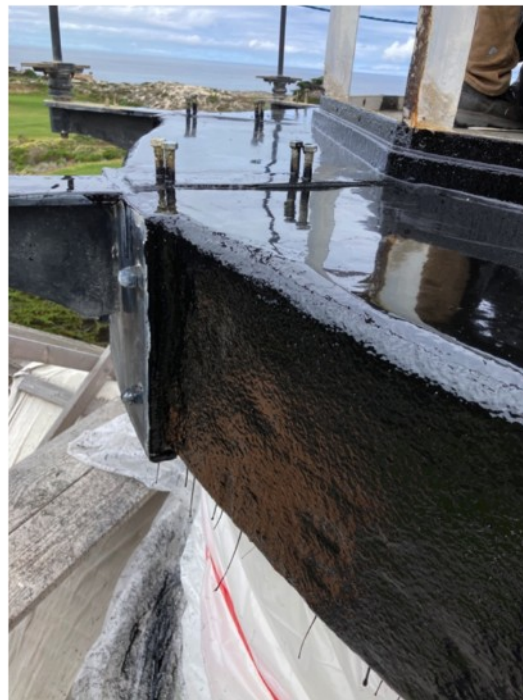
Epoxy coated concrete apron (L) with final coat of black rubberized paint (R)
