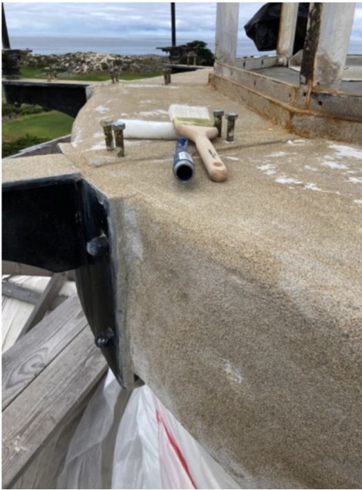
Epoxy coated concrete apron (L) with final coat of black rubberized paint (R)
